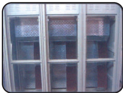
Functional Units Terminal Box Conforms to Form 4B Type 7
